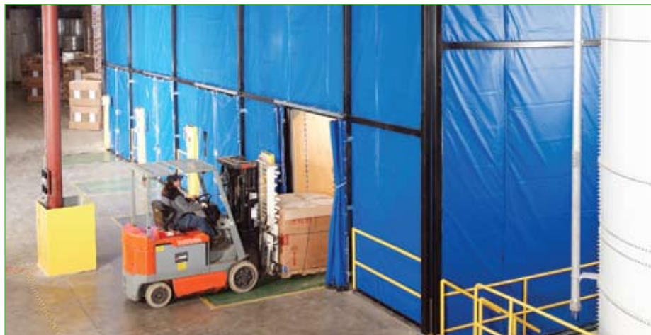
Custom-designed Zoneworks insulated curtain walls enclose the open dock, dramatically improving employee comfort and significantly reducing energy costs in the dock area
